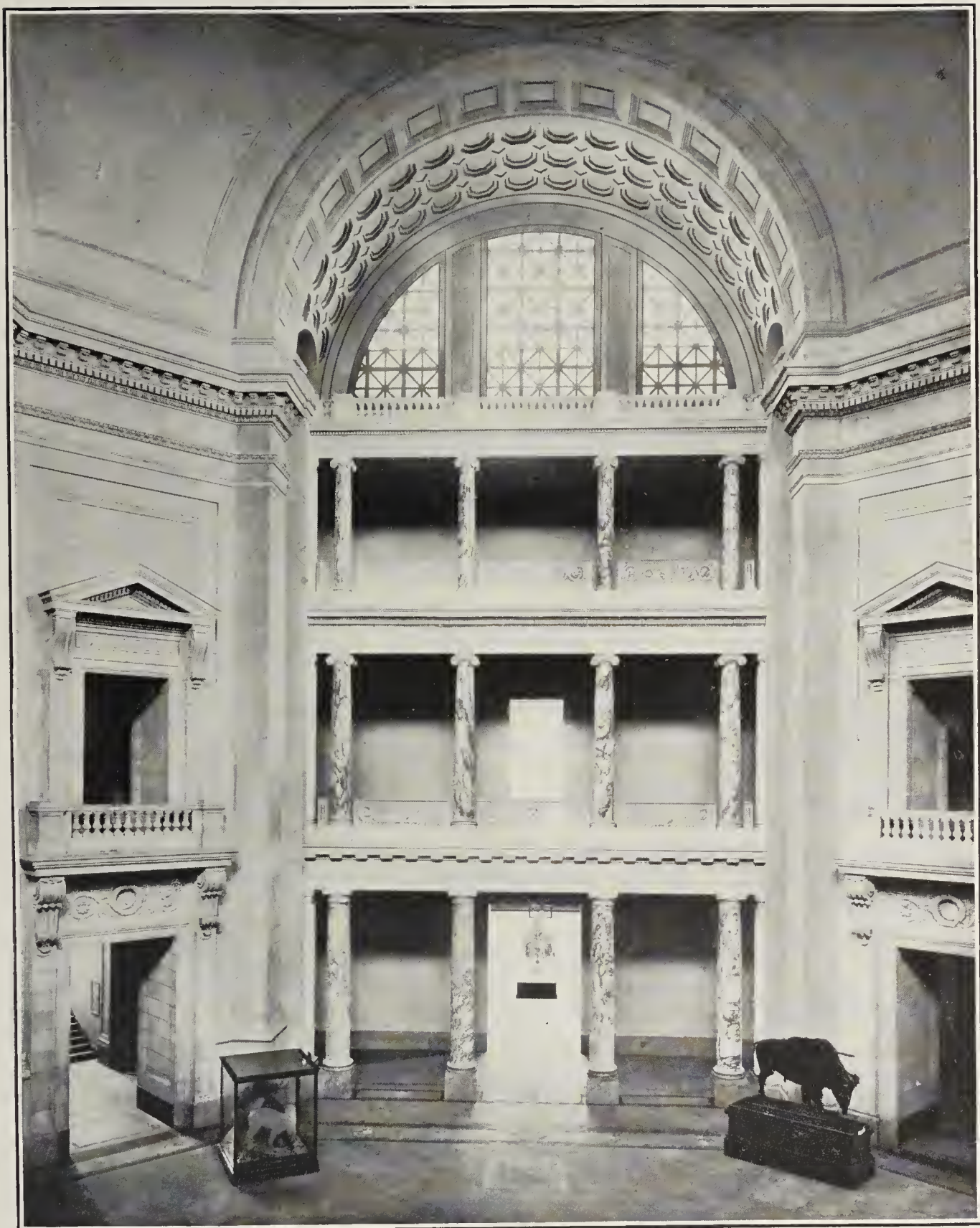
INTERIOR OF THE SOUTH PAVILION AND ROTUNDA TO THE HEIGHT OF THE TOP OF THE GREAT ARCHES, SHOWING THE SCREEN, WALLS, AND CLEARSTORY WINDOW ON THE EAST SIDE, AND PARTS OF THE ADJOINING STONE PIERS.
